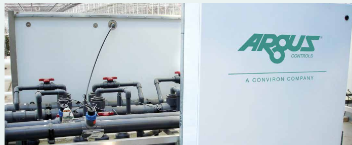
Argus nutrient injection system or control third party equipment for optimal plant growth and operational efficiency.
