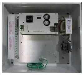
I/O Power Supplies (IOPS) are used on the Titan system to provide power and pass-through communications for the connected devices in an I/O network segment.
